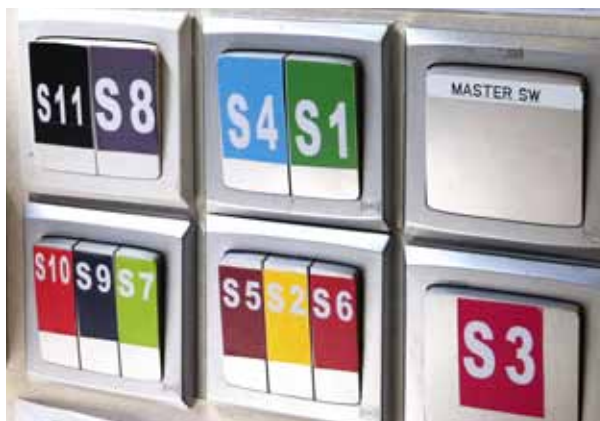
Colour-coded switches to show which office zones they relate.
