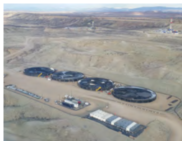
EARL RECYCLING FACILITY, UINTA BASIN
