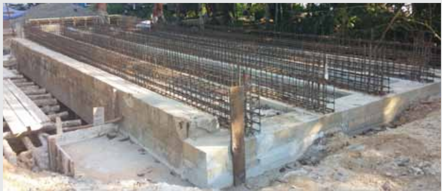
Reconstructing the bridge into a concrete bridge
