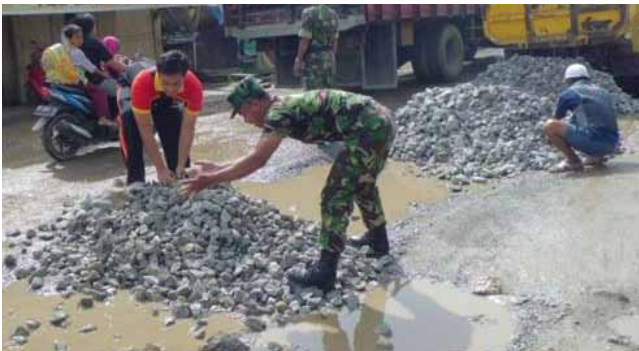
Establish and repairing roads in neighboring villages
