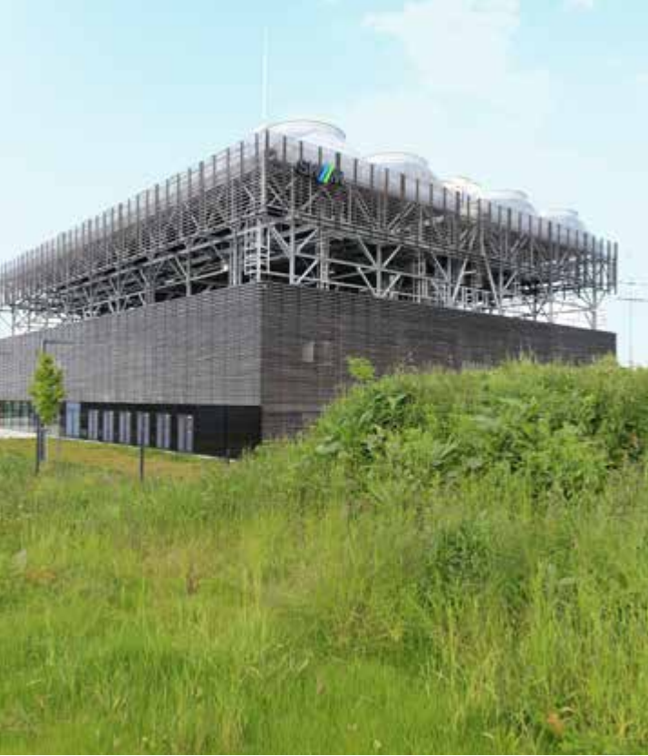
SWM's Sauerlach geothermal plant generates both heat and electricity.
