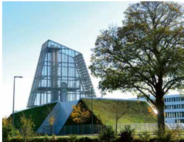
The expansion of geothermal energy is making a major contribution to achieving our climate goals.
