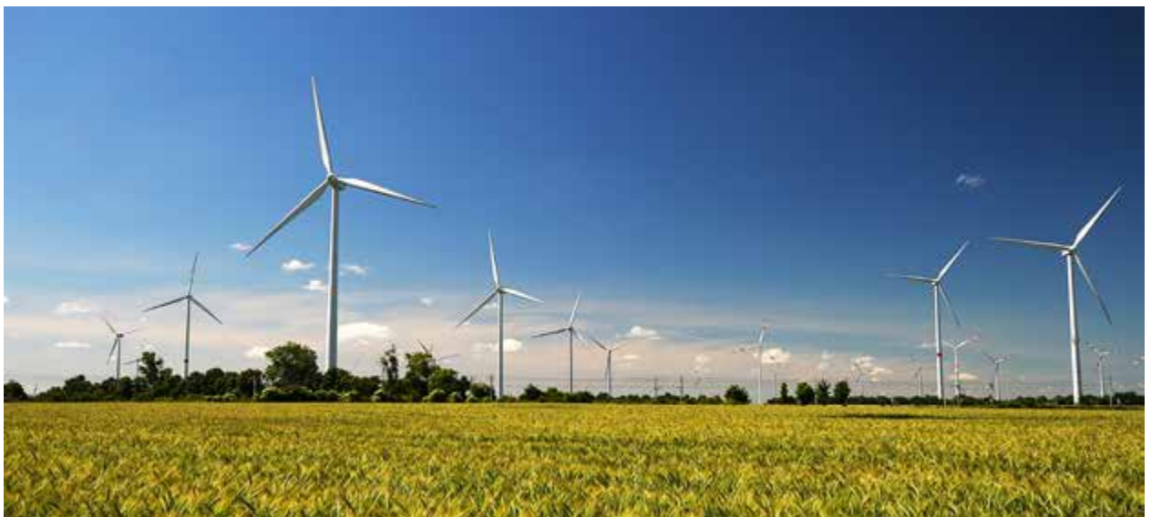
Since 2022, an in-house SWM maintenance team has taken care of the SWM Havelland wind park.
