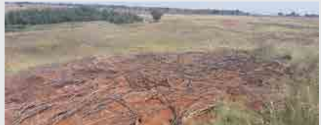
Figure 4: Brush packing placed to reduce water erosion on areas recently covered with topsoil
