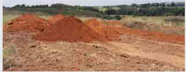
Figure 3: Remediation work on a subsided area in progress
