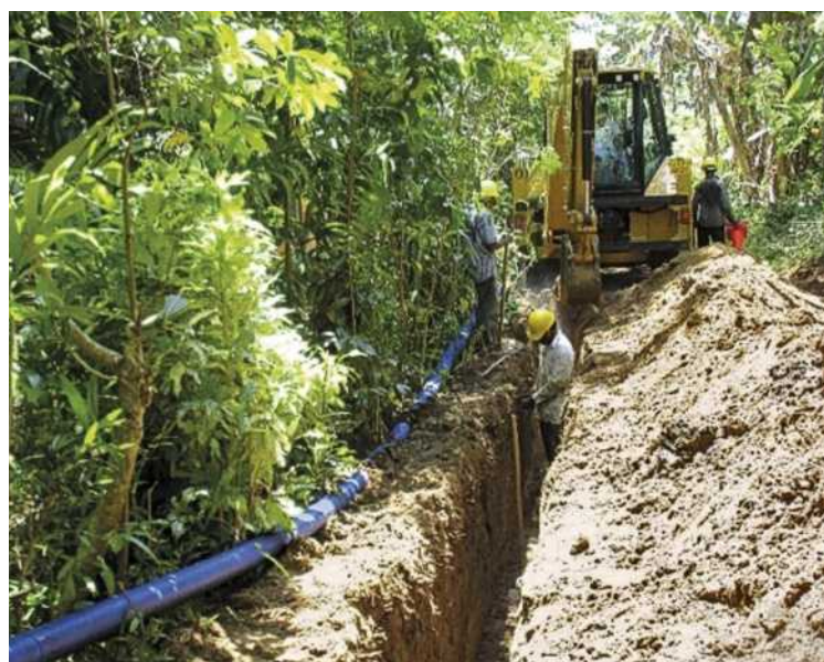
More than 200 000 electrofusion fittings of the ELGEF system are installed in Ampara
