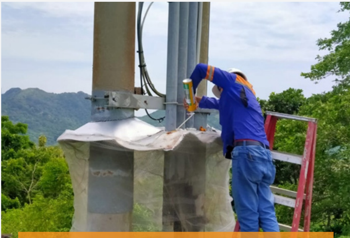
Jaring pencegah fauna memanjat yang berpotensi membunuh fauna dan memadamkan operasional. Protective net barriers to prevent climbing fauna from accessing infrastructure, mitigating risks to wildlife and avoiding operational outages.
