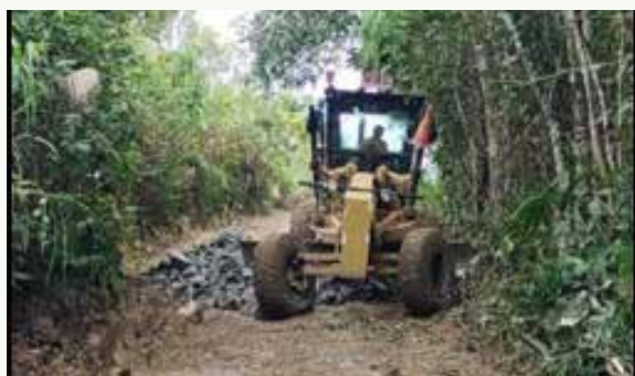
Public Road Improvement
