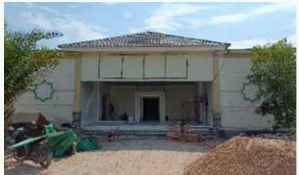
Condition of the STAIS (Sekolah Tinggi Agama Islam Sangatta/Sangatta Islamic College) library after renovation
