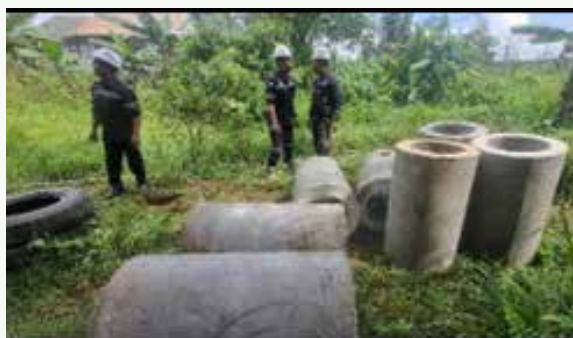
Culvert Instalation Support
