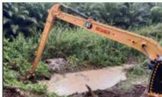
Drainage Culvert Rehabilitation
