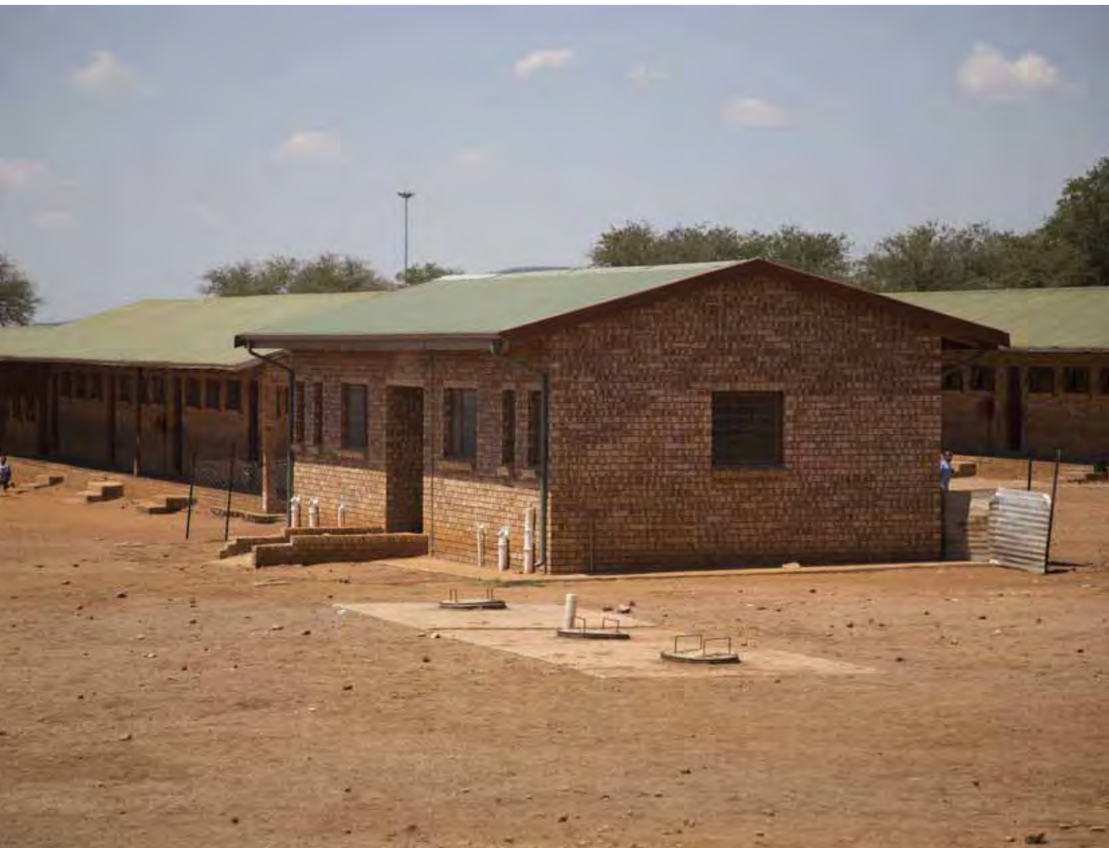
Ablution block built in Phatsima.
