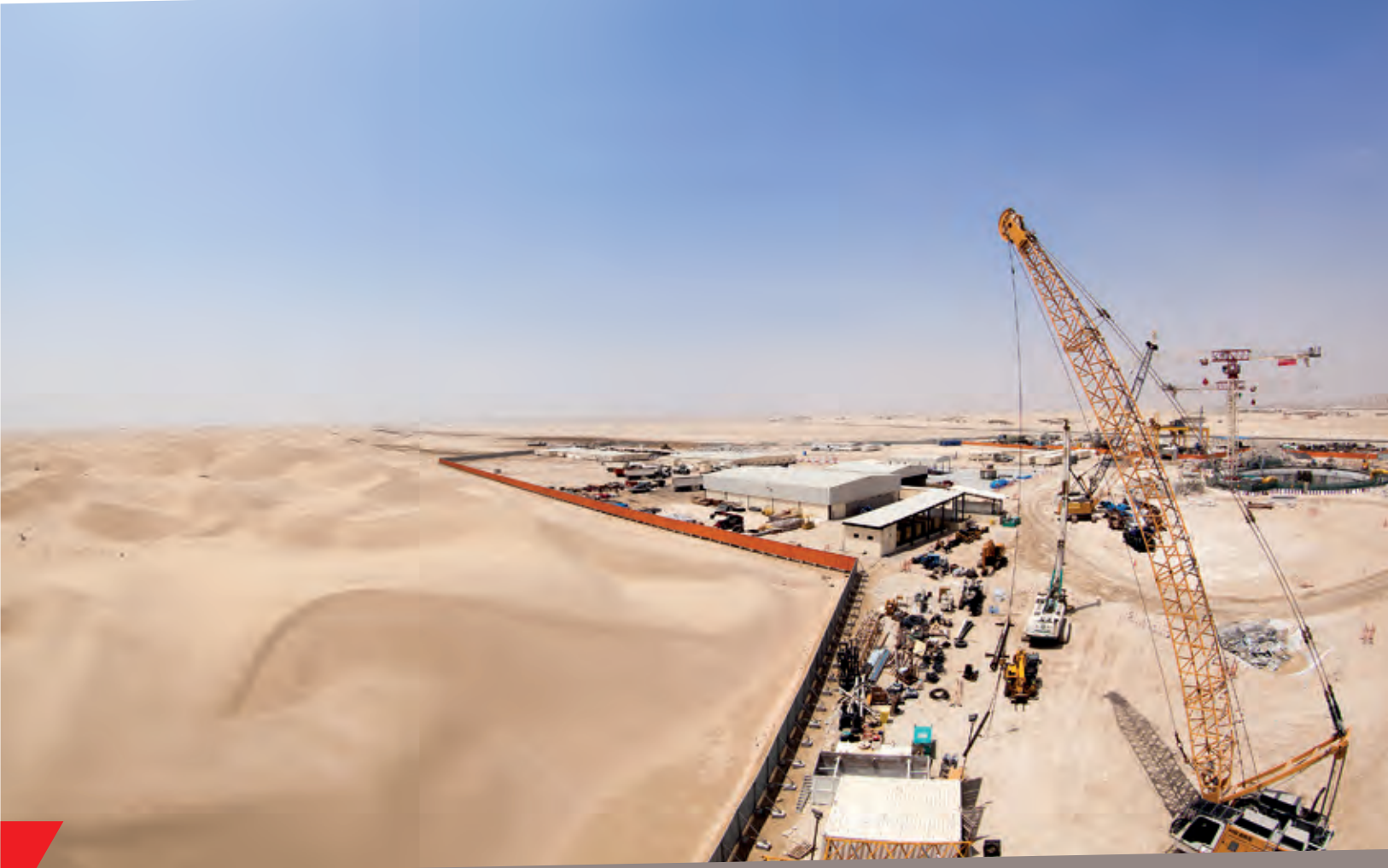
Jobsite for the Abu Dhabi Pumping Station, United Arab Emirates
