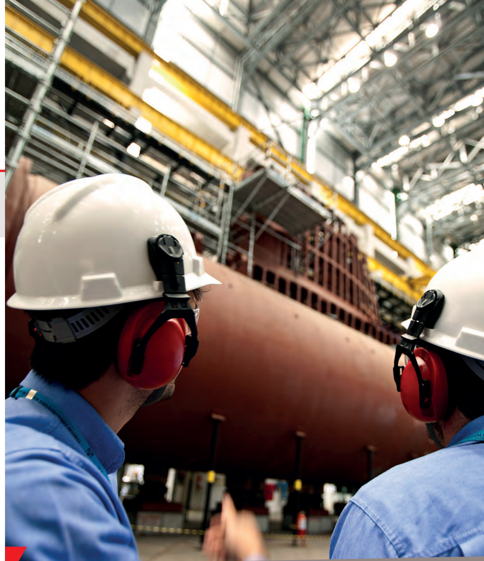
Members Odebrecht Defesa e Tecnologia observe the construction of Brazilian submarine SBR 1 at the Metal Structures Fabrication Unit (UFEM) in Itaguaí, Rio de Janeiro
