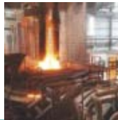
Q-ONE POWER CONVERTERS TO FEED THE ELECTRIC ARC FURNACE
