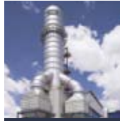
FTP MAIN FANS DRIVE CONTROL
